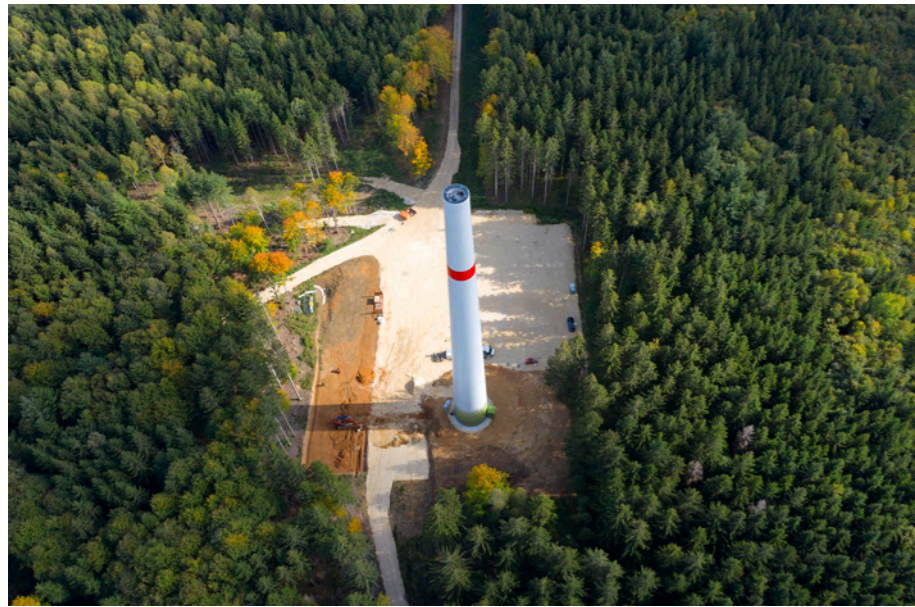
← Steel is used for wind turbine towers, the turbine nacelle, and foundations, as well as for the mounting rack holding the solar modules.
